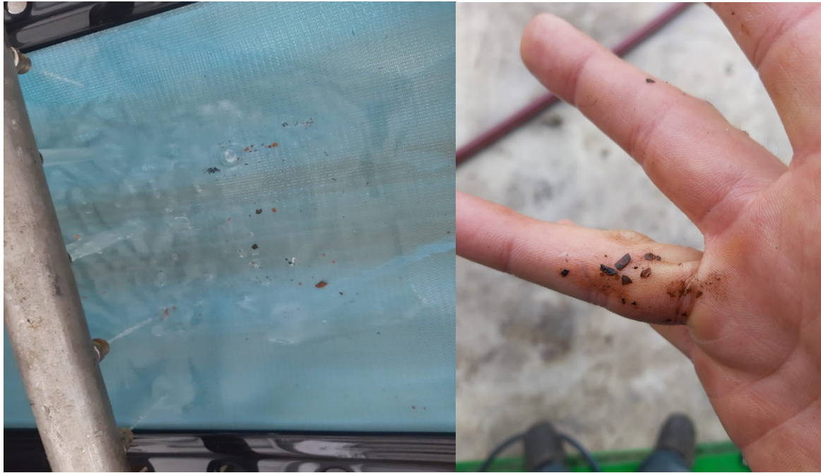
Figure 10 Iron mineral scale collecting on the Z-Filter sock in the area where the sock is cleaned by a high-pressure water spray. The outer two spray nozzles in the left photo appear to be partially blocked.
